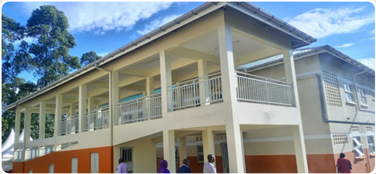
The commissioned structure
