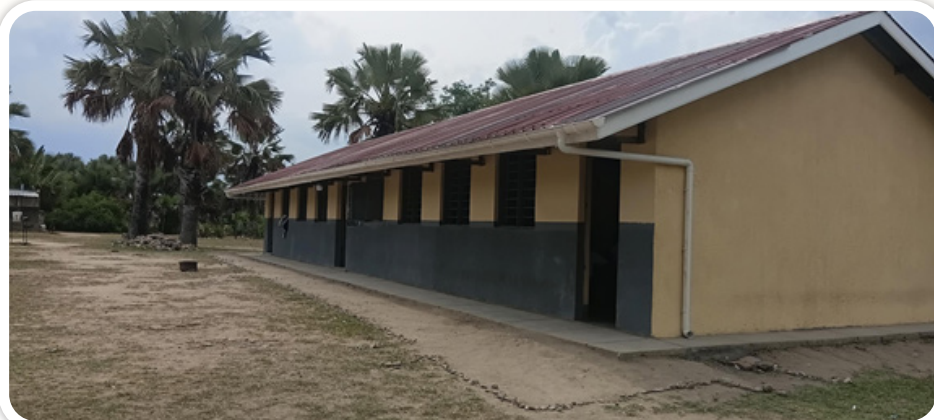
Renovated 2 classroom block with admin office at kamuhigi Primary School
