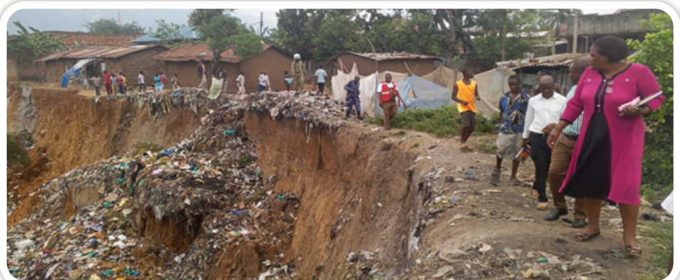
Some Disaster committee members inspecting a disaster prone area at Kisenyi, Bundibugyo town council. (Photo by Tibesigwa Rajab CO Bundibugyo)
